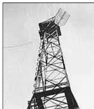
The studio tower, clearly showing the "beam-bender"
